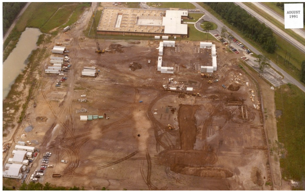
Arial photo of current Unit 5 and 1992 expansion underway
